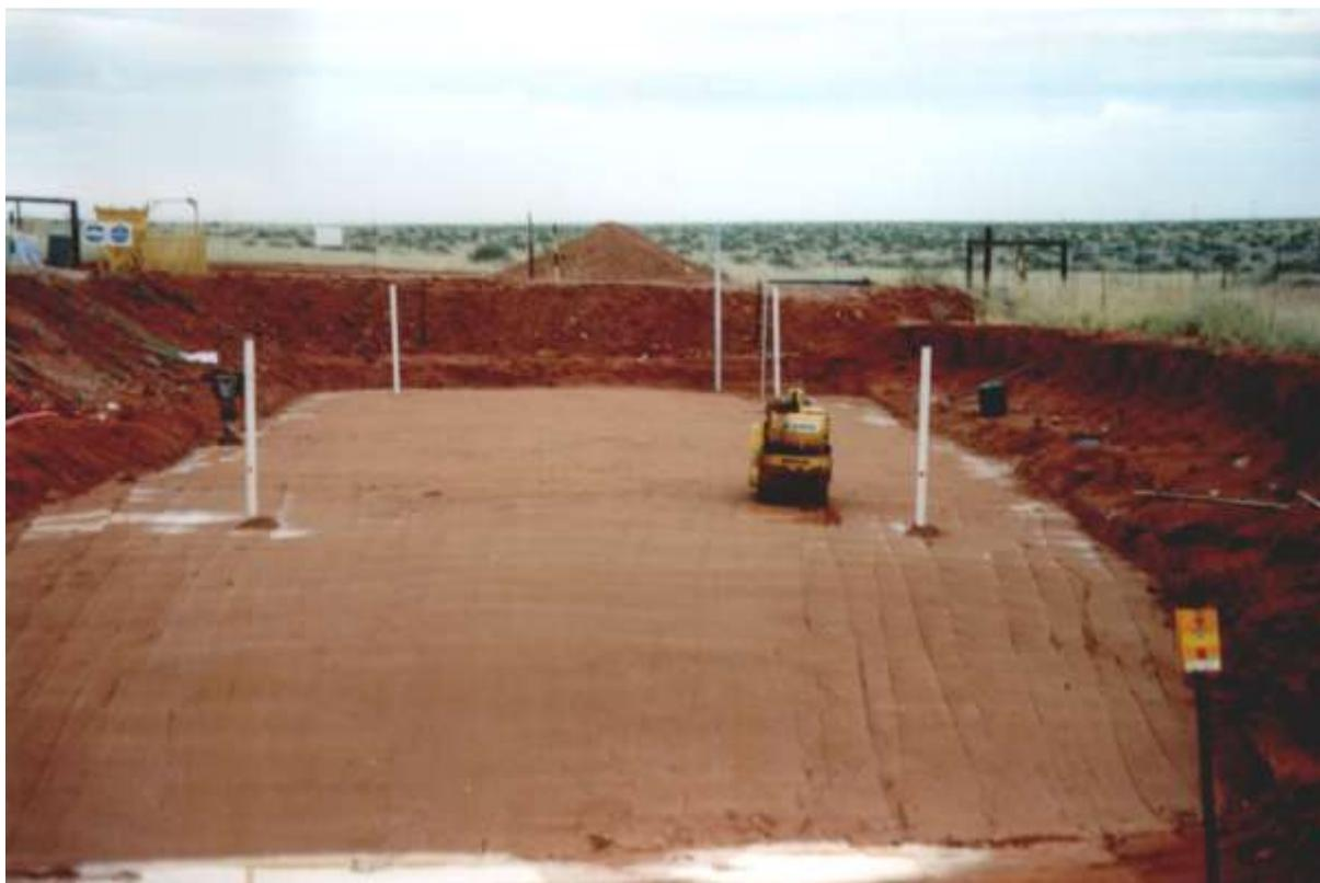
**Figure 7: Capping of near surface disposal trench**
